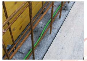
The hose has to be well set on the cold joint and has to be fastened with hose clamps at **approx. 15 cm** distance (depending on surface of the concrete of the construction joint).
